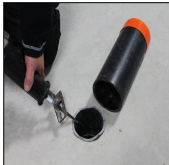
After concrete poured cut pipe flush to floor
