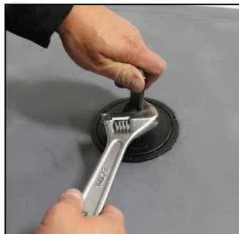
After solvent cement sets, tighten plug flush to floor
