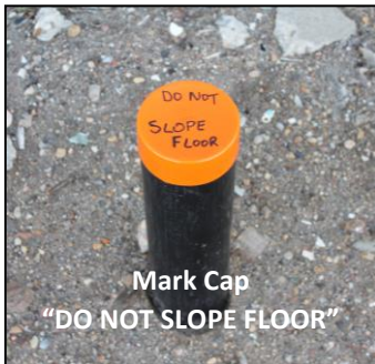
Mark Cap "DO NOT SLOPE FLOOR" Bring pipe up above finished floor height and cap
