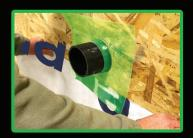
Overlap building wrap over seal (install complete).
