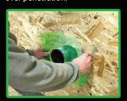
Slide building wrap under bottom of seal.
